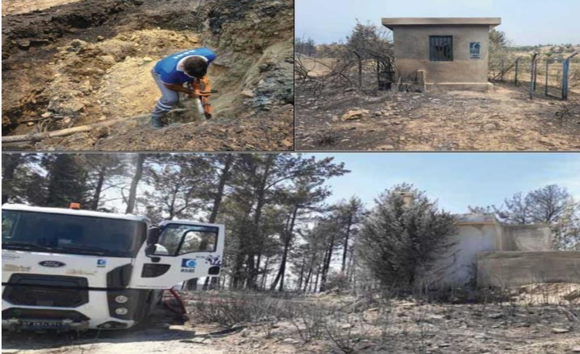
Figure 2: Situation of Affected Infrastructure After Wildfire Disaster (Images of Drinking Water Network, Water Storage Tank, Pumping Stations)
